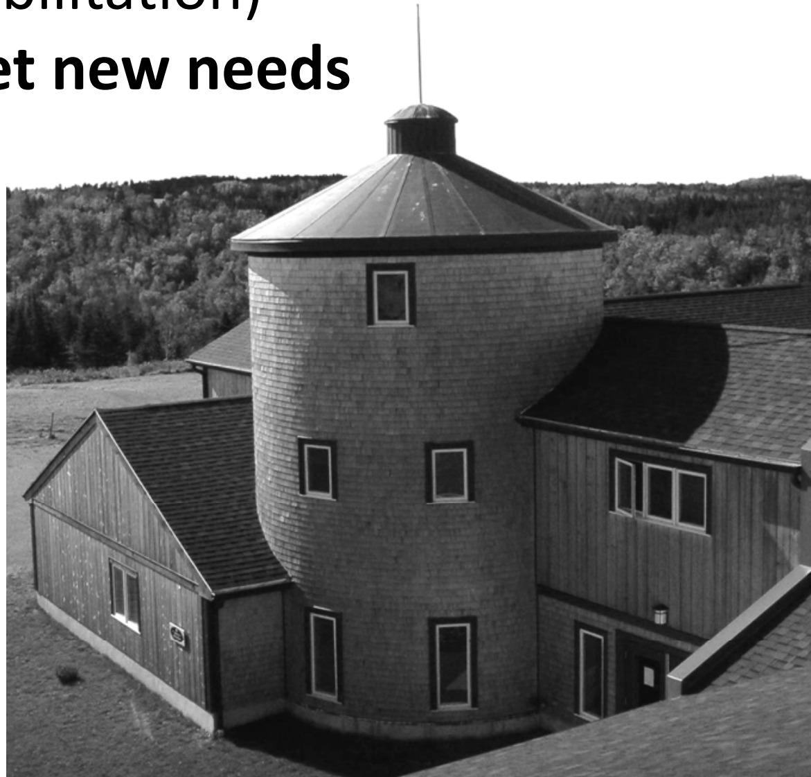
The Ross Creek Centre for the Arts Canning, Nova Scotia
