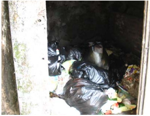
Picture 2.2 Waste Storage Room in CongDoan Hotel
