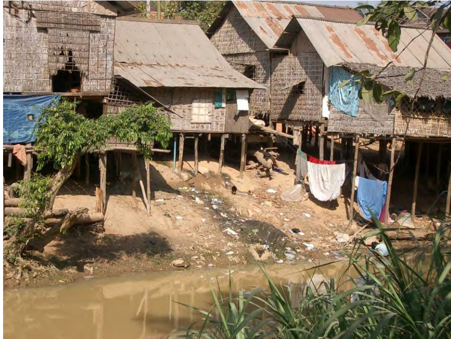
Figure 4. Houses encroaching on the riverbank; waste along the riverbank
